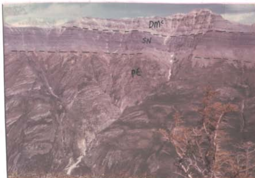
Plate 9. Sentinel Range, stratigraphic section north of Toad River Bridge (Mile 437 1/2 on the Alaska Highway). This is the type area of the Nonda Formation. Note gabbroic dykes cutting the Pre-Cambrian rocks and the angular unconformity between the Pre-Cambrian and Nonda strata.
