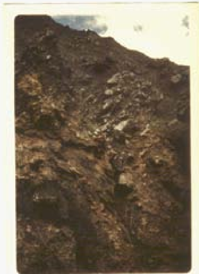
FIG. 1 Fault breccia of Unit 1. Block on lower left (S) is about 2 feet wide.
