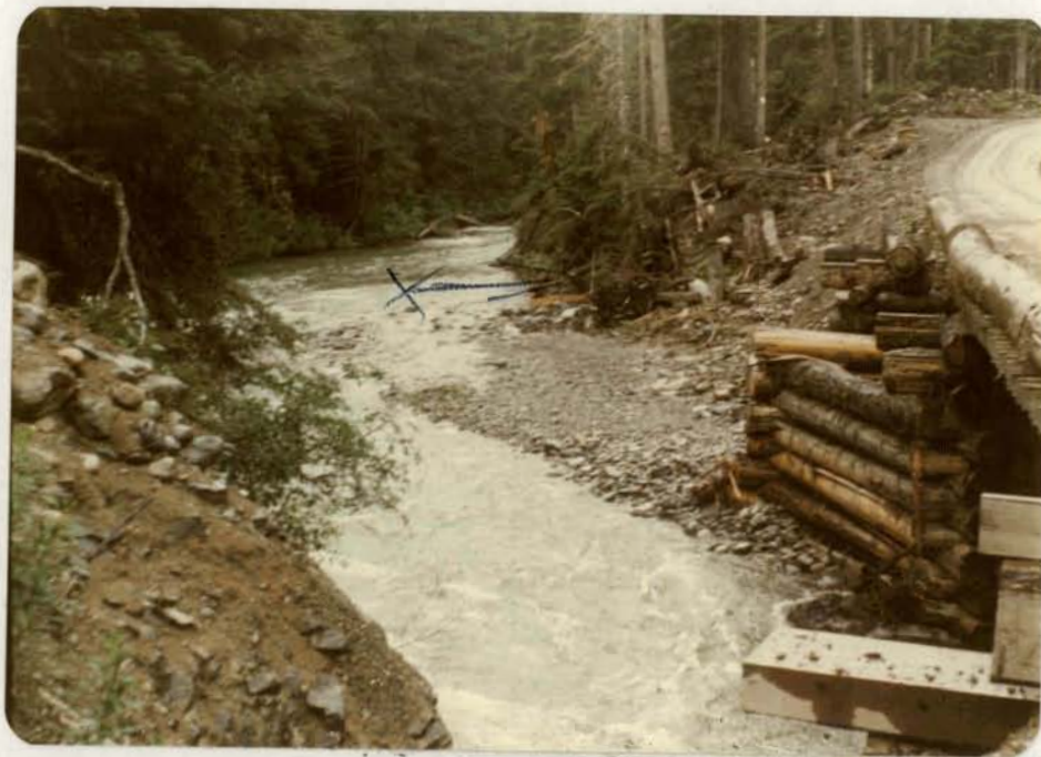
Fig 4 a. CanCel Bridge, looking south. X marks the locality sampled.
