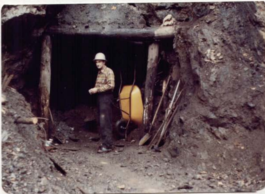
Plate V. Clearing Silver Adit Completed.
