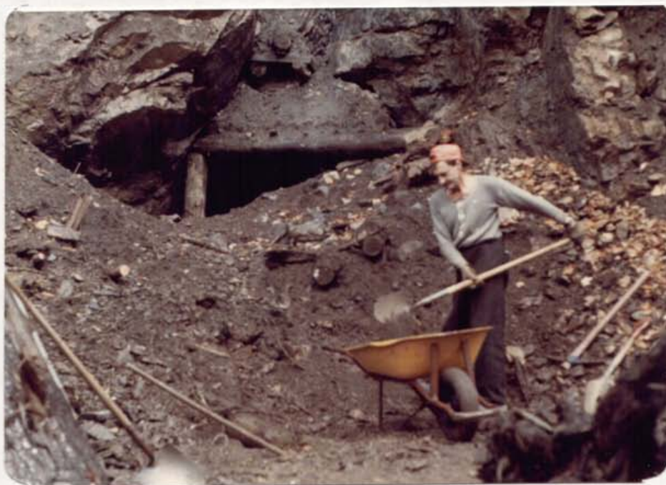
Plate IV. Clearing Operation at Silver Adit Begins.
