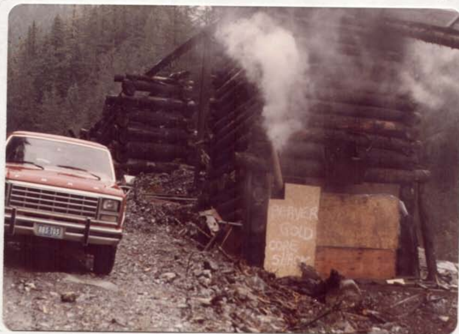
Plate VII. Core Shack in Old Ore Bin.
