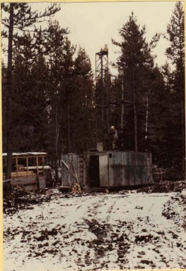
PHOTOGRAPH 1 : LONGYEAR SUPER 38 DRILL COLLARED ON HOLE 84-2.
