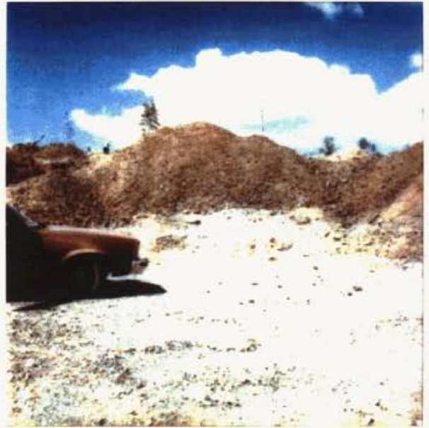
VIEW OF TRENCH RUBBLE LOOKING NORTH
