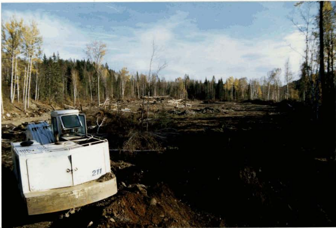
FREEGOLD RECOVERY'S BACKHOE WORKING ON TAILING PONDS, TRENCHING AND STRIPPING
