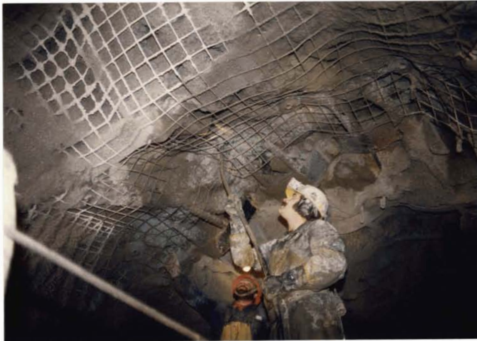
INSTALL CEMENT FONDU INTO DRILL HOLES (ROCK BOLT TEST)
