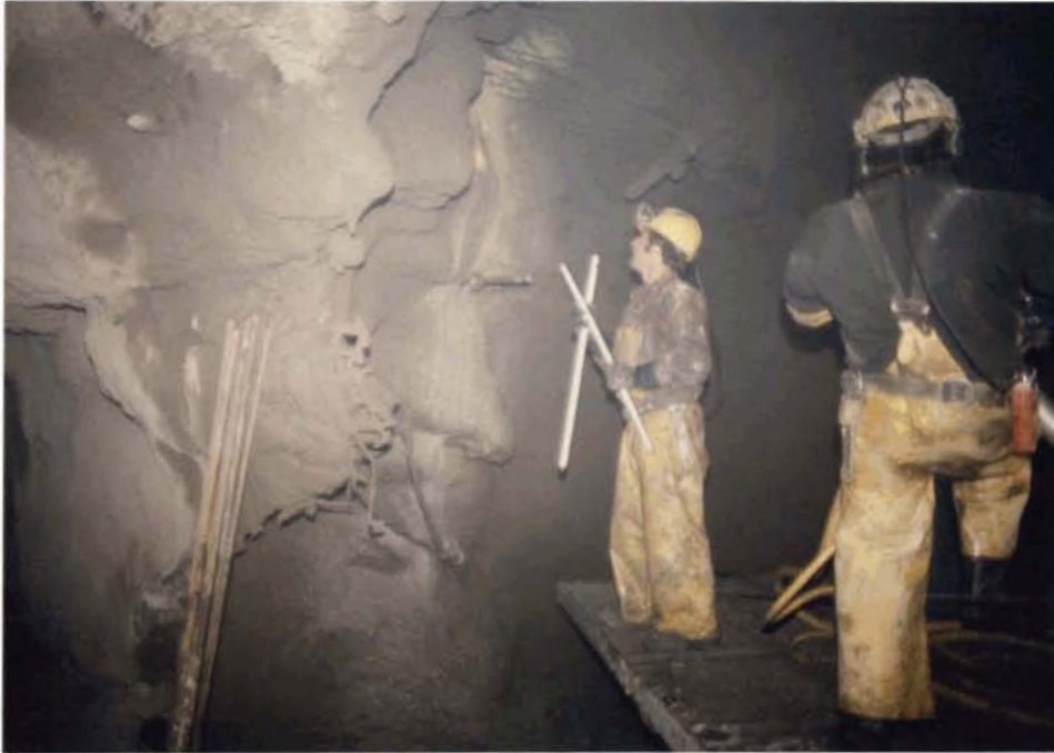
INSTALLING RESIN CARTRIDGES FOR DYWIDAG ROCK BOLTS
