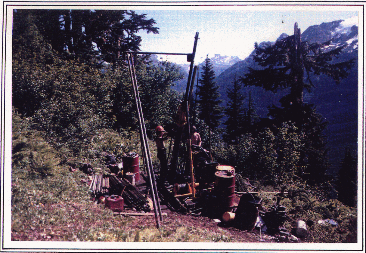
Plate 1: Hydro-Core Diamond Drilling Rig
