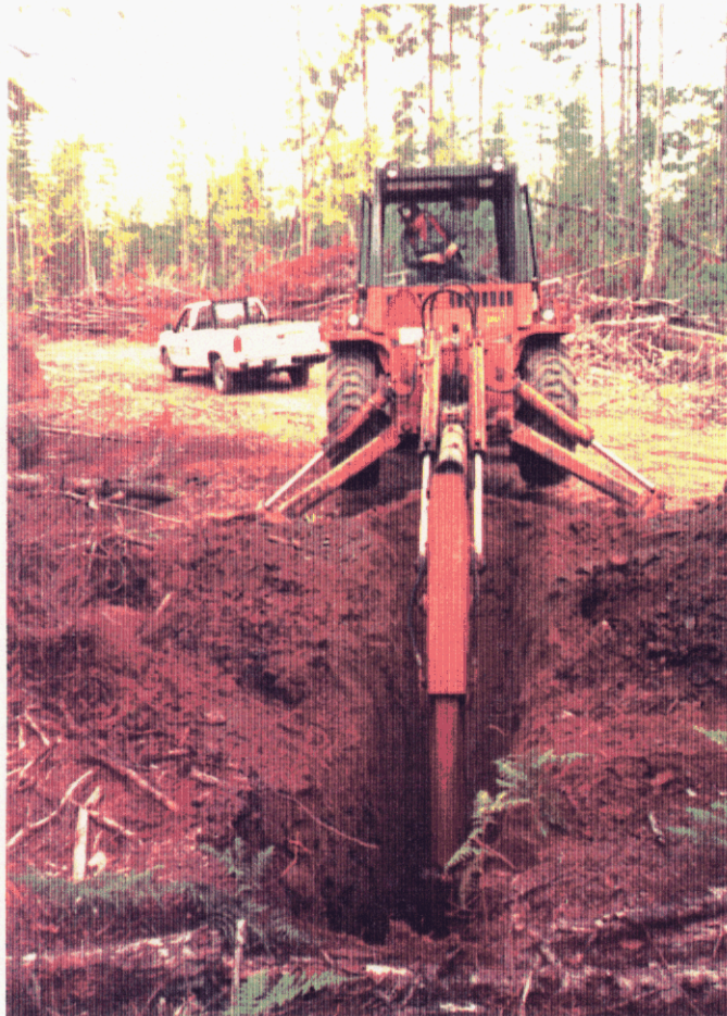
Photo #1: Backhoe Excavator
