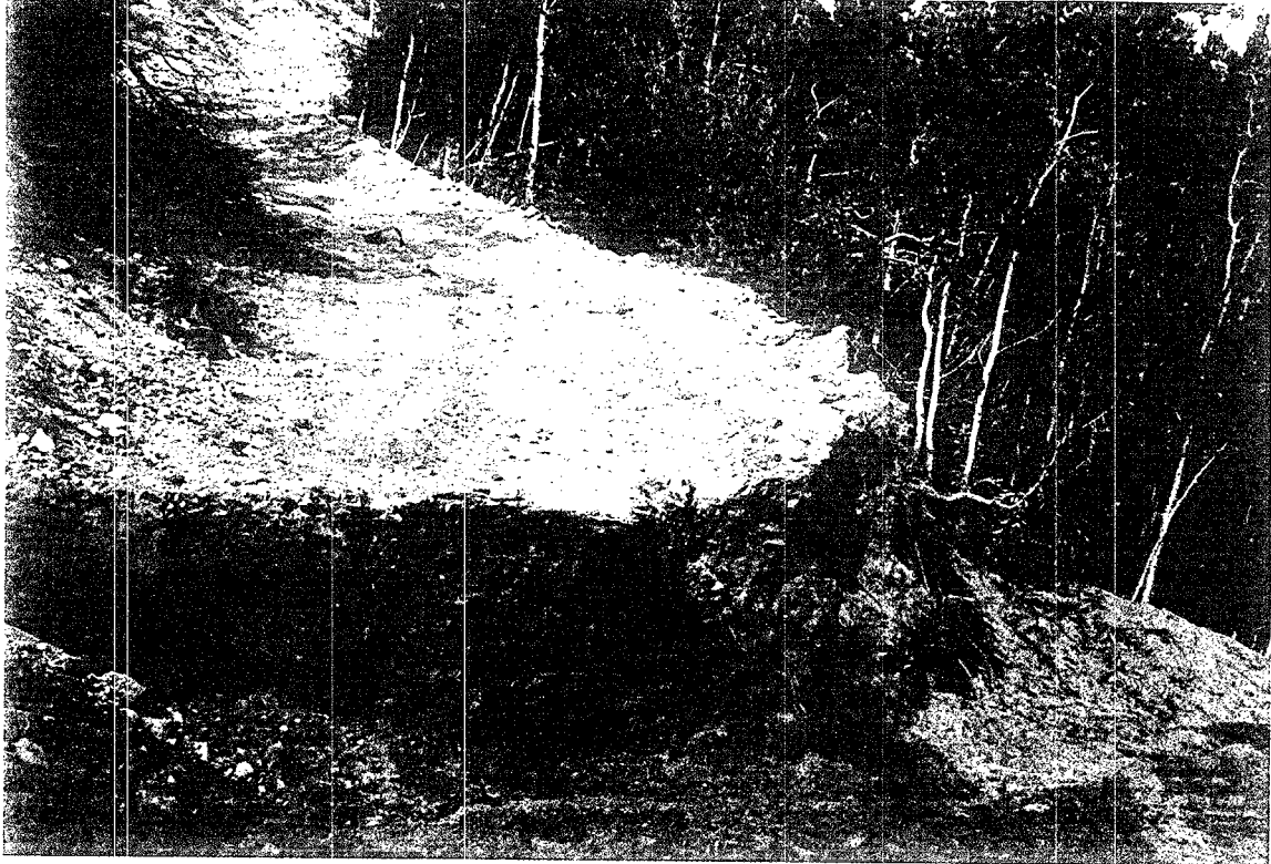
Photo 15 Access Road: Cut across main access road.
