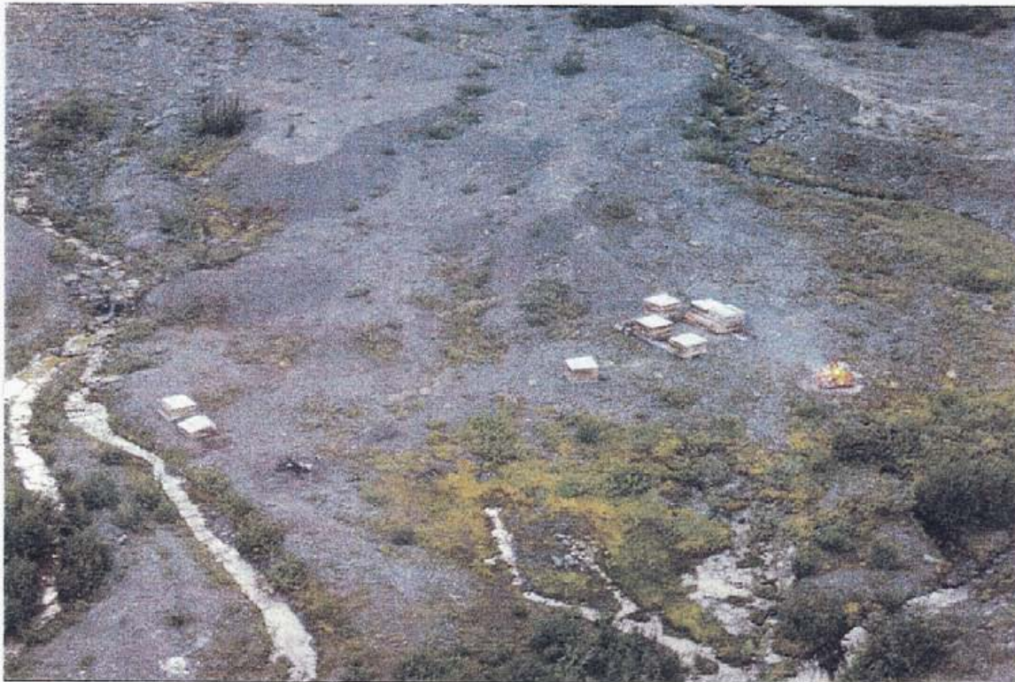
Photo 1 Todd Creek South Camp after reclamation.
