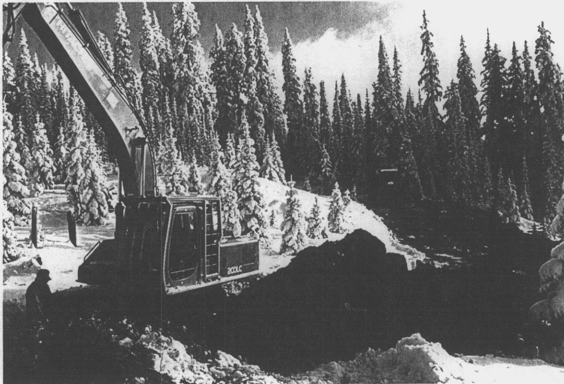
Pacific Rim Equipment performed trenching along pre-existing roads to avoid disturbing vegetation, all trenches were backfilled and levelled. Immediately behind backhoe is sample 9,462-63 which returned 13.2 ft.(4 m.) of 0.285 oz/t Au (9.77 g/t Au).
