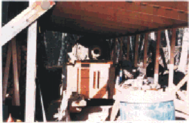
DAUL MILL - INTERIOR VIEW
