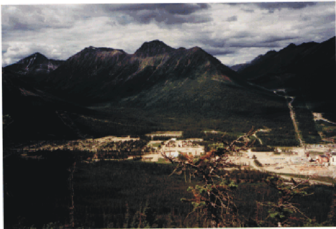
FIGURE 5. The Cassiar asbestos mill site, looking north from the D-Zone area of the Southern Block.
