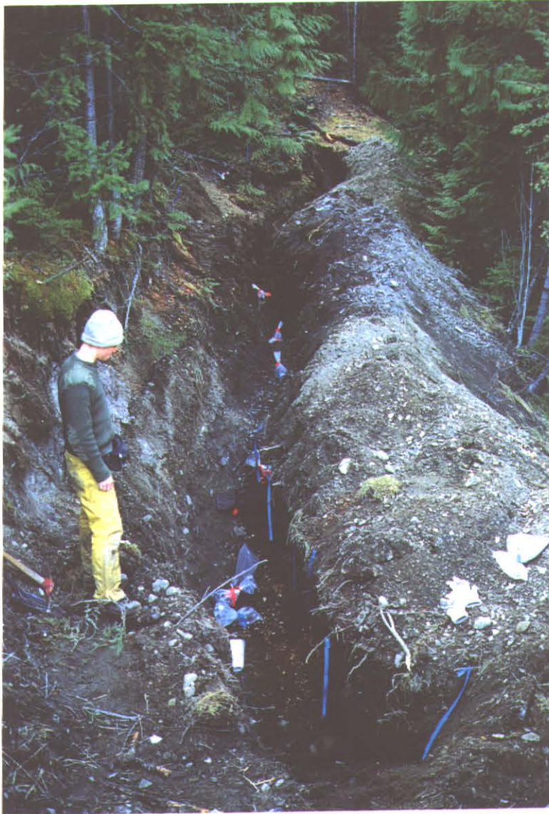
THE BULLDOZER TRENCH SHOWING TRENCH 3 Photo # 1
