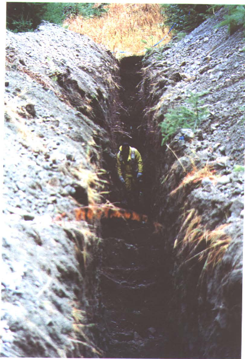
THE BULLDOZER TRENCH SHOWING (TRENCH 4) Photo # 2
