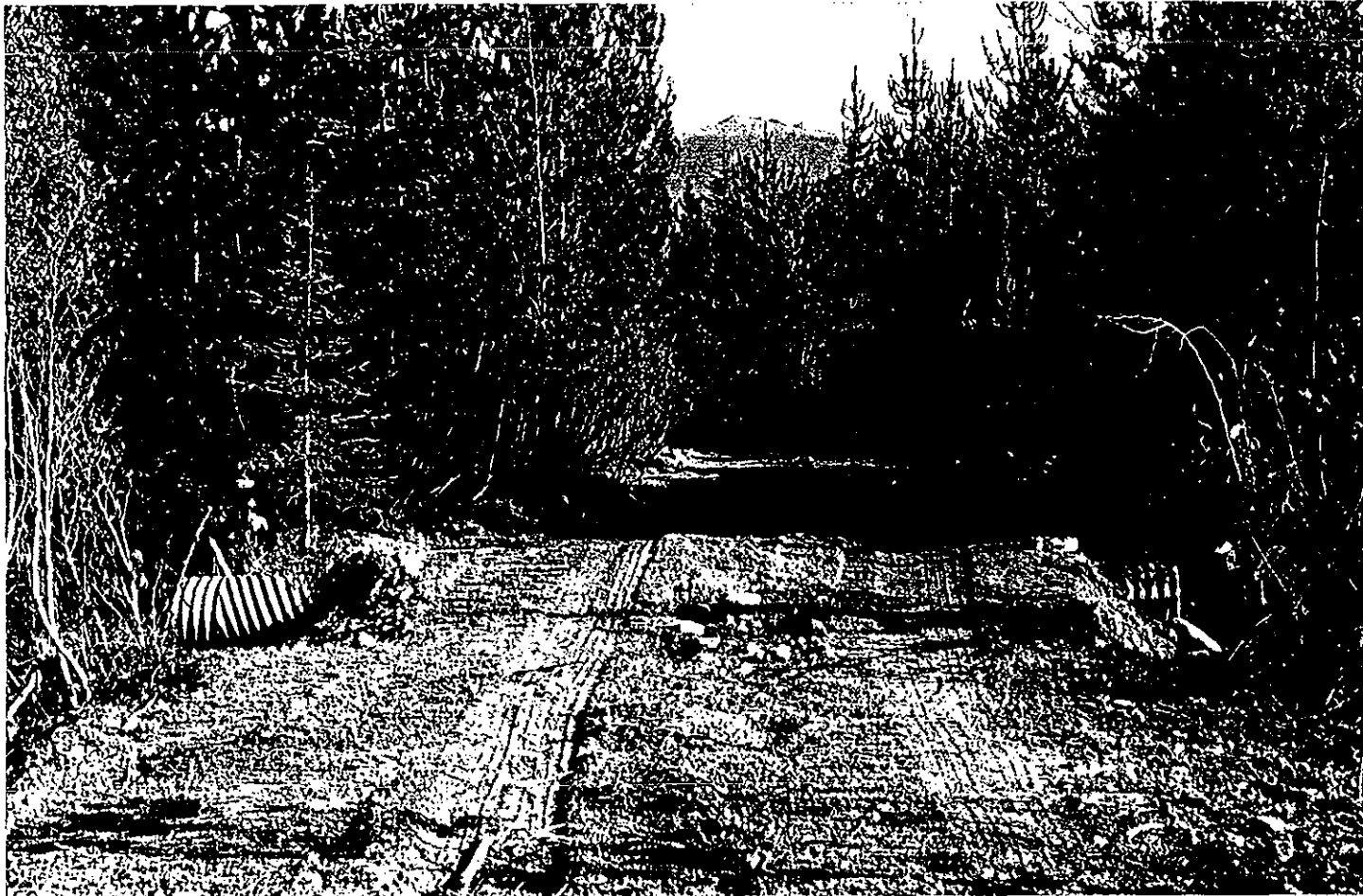
Plate 4. Rehabilitated access road (Grid 5 area)
