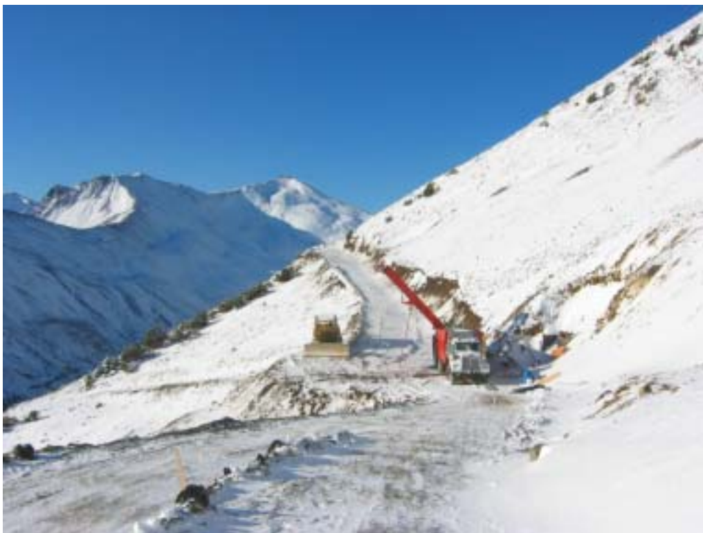
Photo 5. DDH 02-14 at Upper Adit Portal
