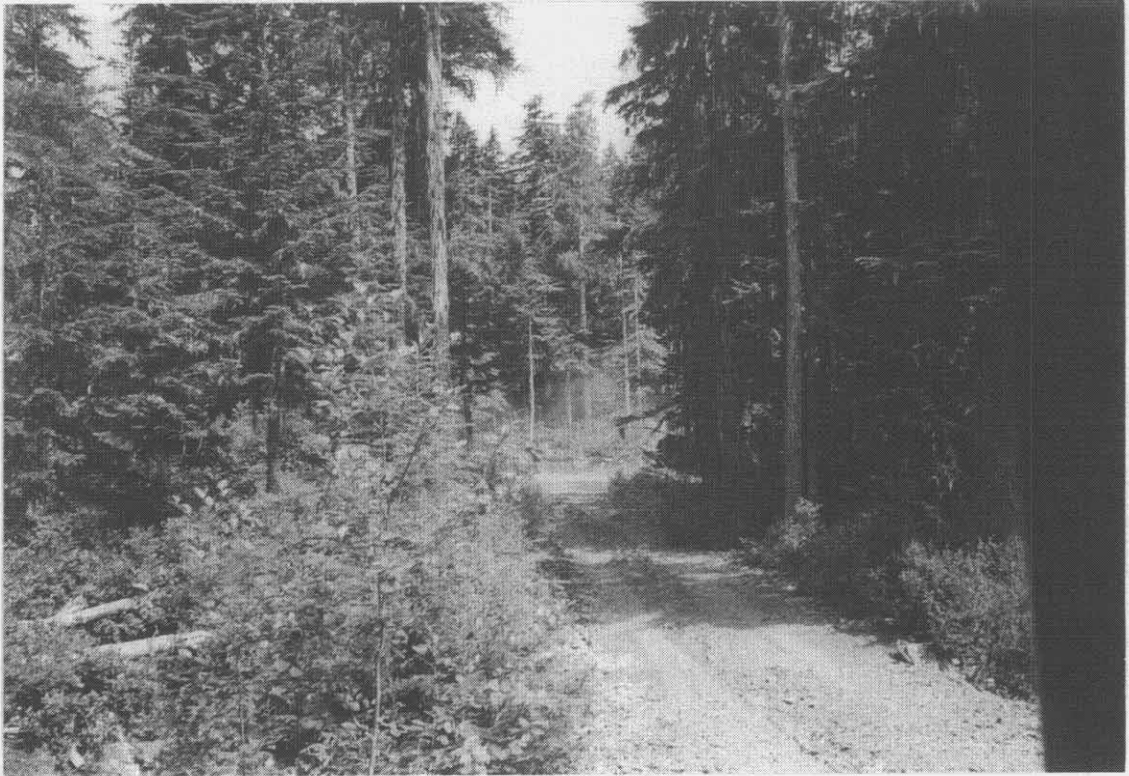
BLAZE 2 CLAIM- ACCESS ROAD IMPROVEMENTS (2002), LOOKING NORTH
