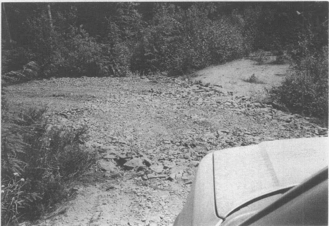
BLAZE 2- ACCESS ROAD IMPROVEMENTS (2002), LOOKING NORTHEAST
