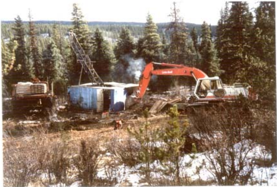
Plate 10: Drill hole 99-7 (view showing equipment, May, 1998)
