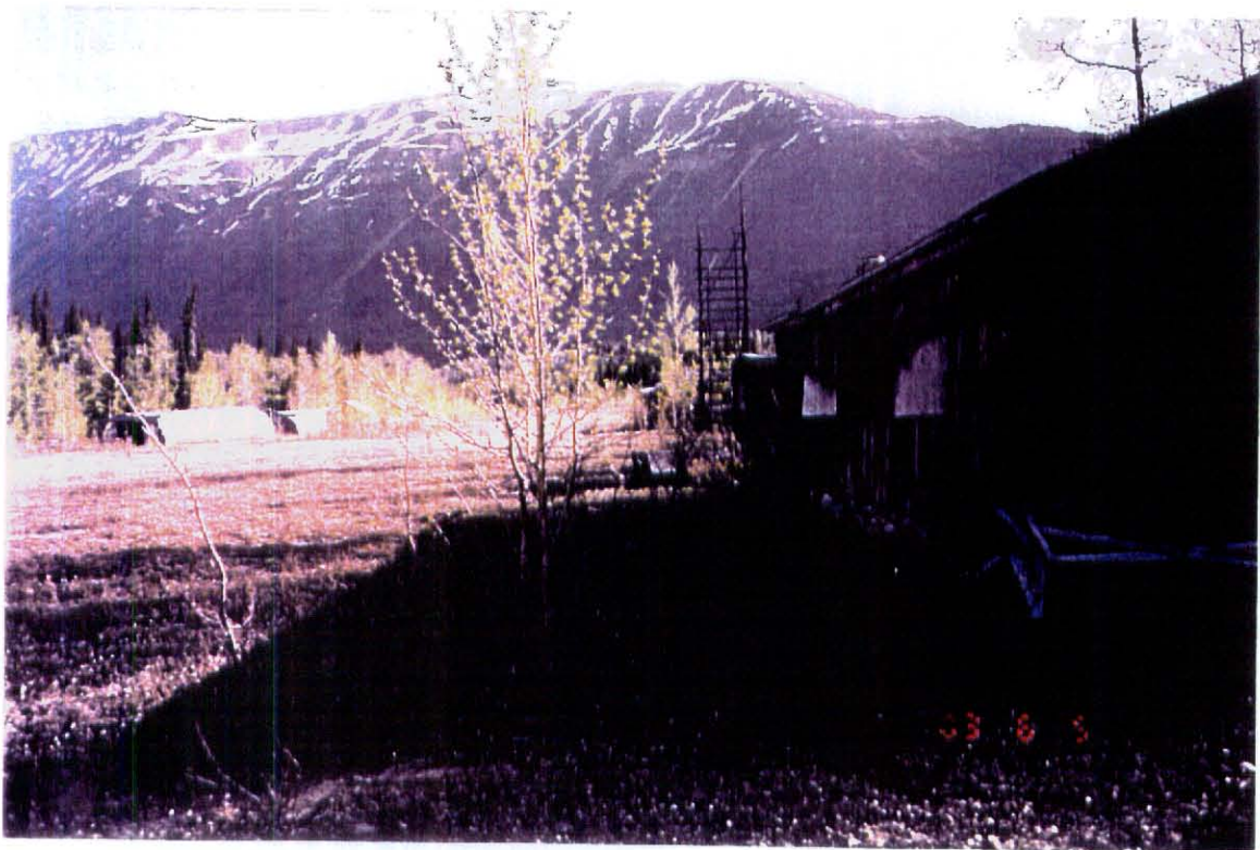
GENERAL VIEW OF CAMP OPEN SPACE & BUILDINGS
