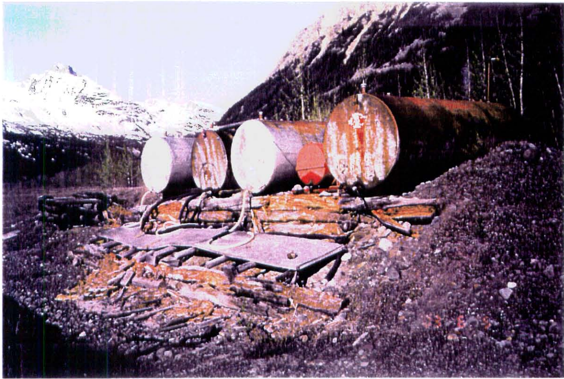
CAMP FUEL STORAGE TANKS & RE-FUELING BAY
