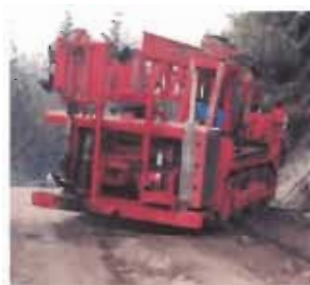
Drill on-site in the Pearson project area at Pope's Nose Showing
