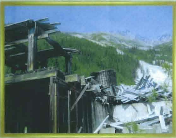
MILL BUILDING AT 1,200 LEVEL PORTAL (1,280 m ELEVATION).
