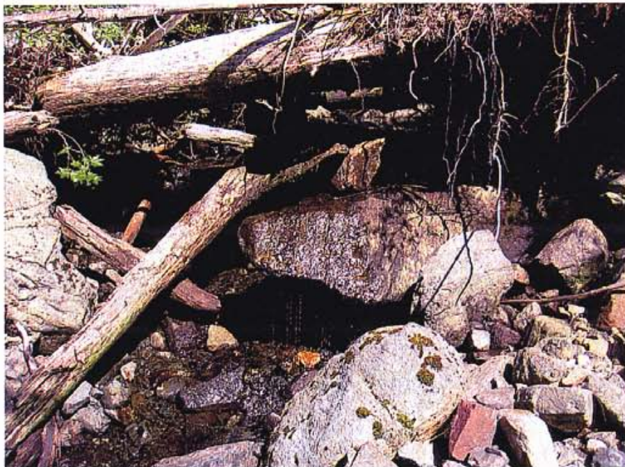
Photo 11 Site 3, looking upstream.
