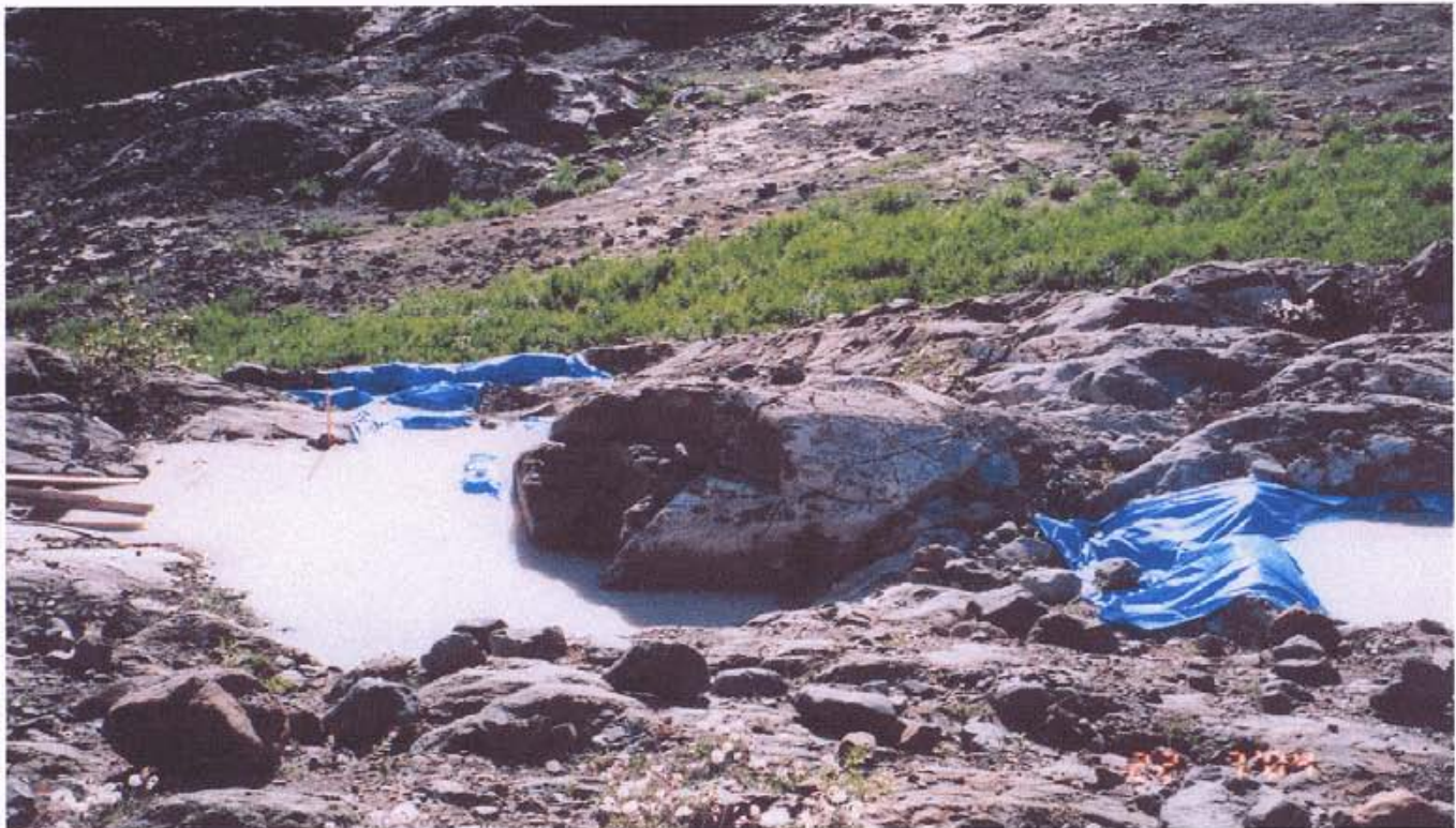
PHOTO 9: AREA OF DDHSZD04-04: LOOKING SOUTHWEST AT UPPER SUMP PONDS WITH TARPS IN PLACE.
