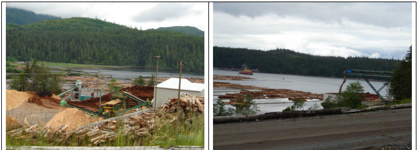
Northland Power's woodchip and barging facility at Beaver Cove.
