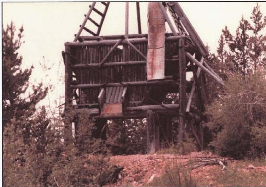
Figure 16 Original Headframe of Lucky Todd Shaft
