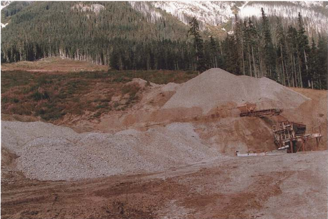
Photograph 4 – Wash plant under construction.
