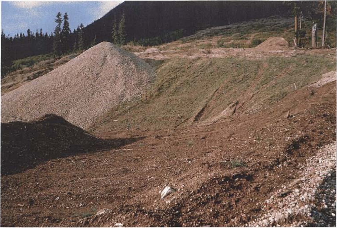
Photograph 3 – Area previously planted for erosion control (centre) , additional soil stockpiled (foreground).
