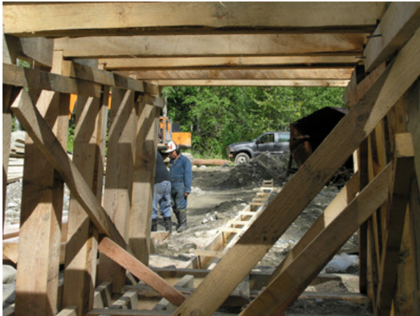
Cross bracing is installed to keep the sets square.
