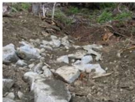
Ditch Outlet Armouring
