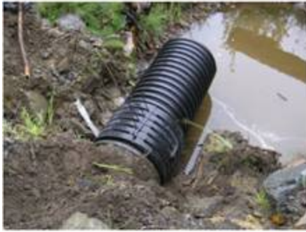
Culvert Inlet Extension
