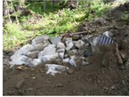
Culvert Outlet Armouring
