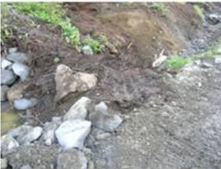
Culvert Inlet Ditch Block and Armouring
