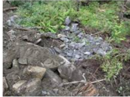
Culvert Outlet Armouring
