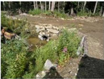
Culvert Inlet Armoring
