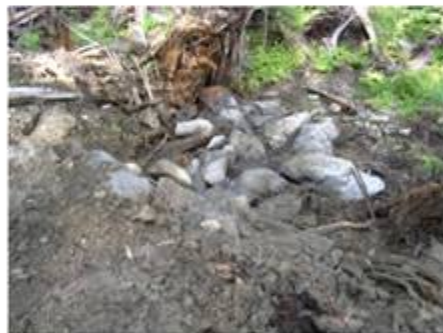
Culvert Outlet Armouring
