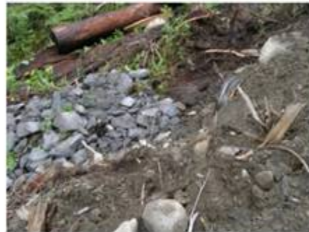
Culvert Outlet Armouring
