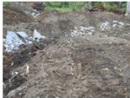
Ditch Outlet Armouring
