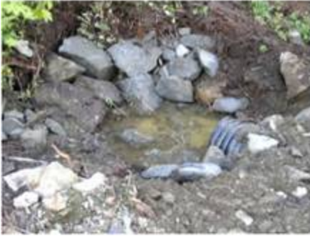
Culvert Inlet Sediment Trap and Armouring
