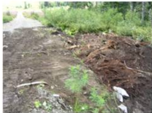
Ditch Clean-out and Armoring
