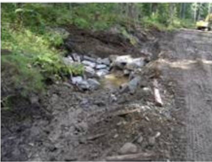
Culvert Inlet Sediment Trap and Armouring
