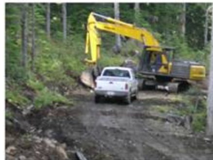
Ditch Clean-out Slope Contouring
