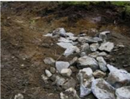
Inlet Ditch Block and Armouring
