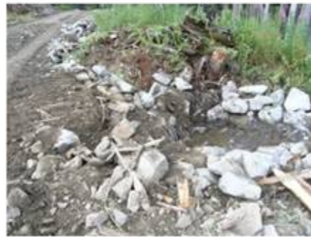
Culvert Outlet Armoring
