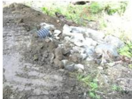
Culvert Outlet Armouring
