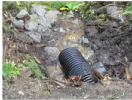
Culvert Outlet Extension
