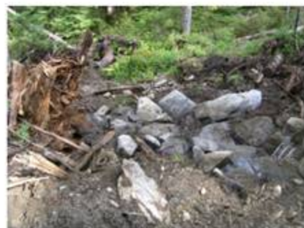
Culvert Outlet Armouring
