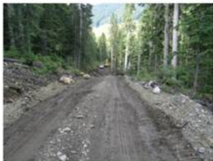
Ditch Clean-out Slope Contouring
