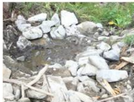
Culvert Outlet Armoring
