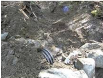
Culvert Inlet Ditch Block and Armouring
