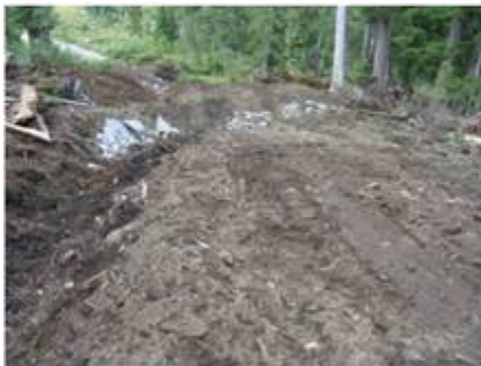
Ditch Inlet Armouring
