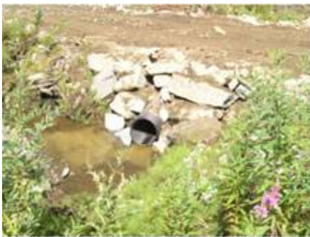
Culvert Inlet Armoring
