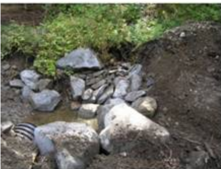
Culvert Inlet Ditch Block and Armouring
