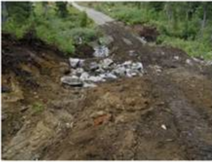
Inlet Ditch Block and Armouring
