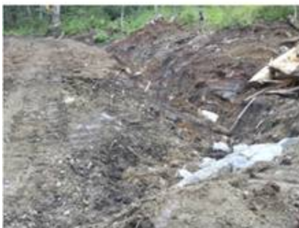
Ditch Inlet Ditch Block and Armouring
