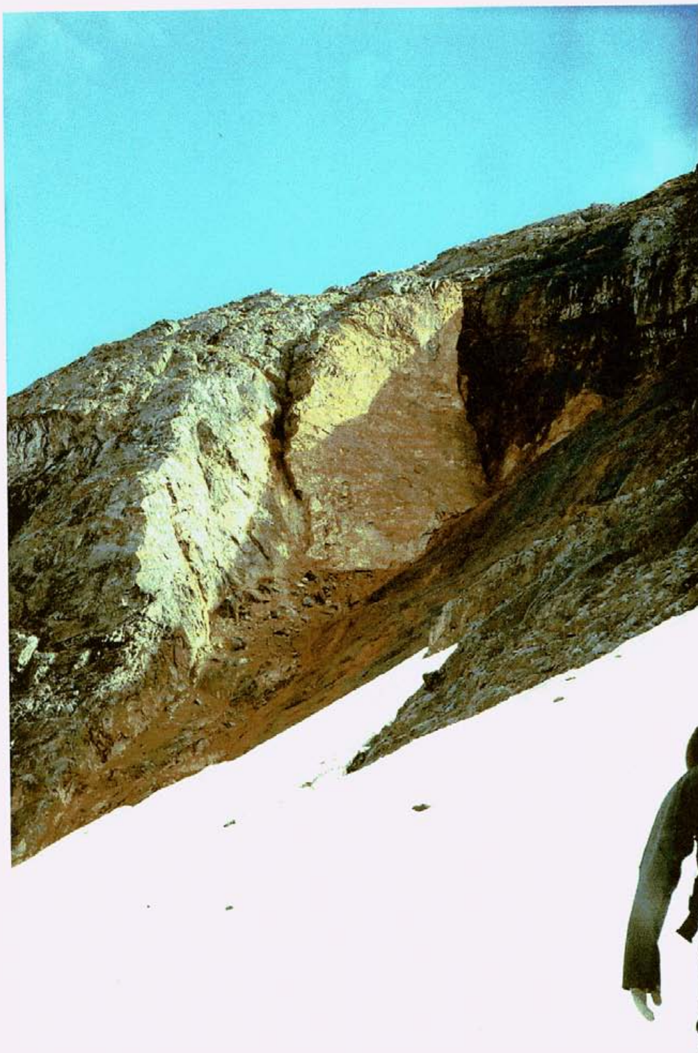
Photo 1350009: Close up of previously mentioned fault bounded slide chute, containing a large, loose, hanging block. The most prominent fault cutting the chute trends north-south, and dips steeply.
