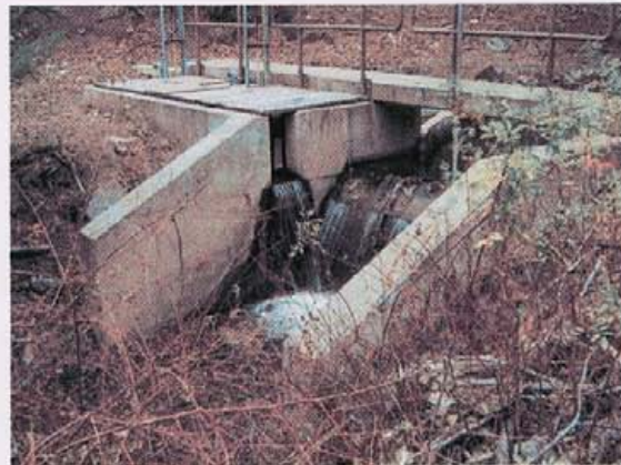
Figure 3. Flow control structure on McGillivray Creek.
