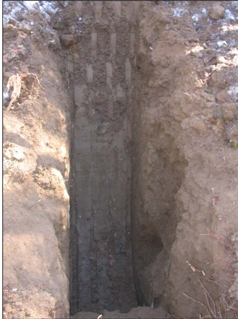
PHOTO #4 – TP06-19 Near WMF South Embankment
