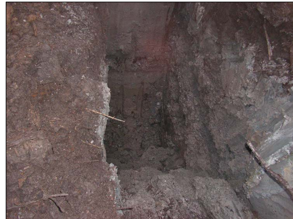
PHOTO #6 – TP06-24 at Plant Site
