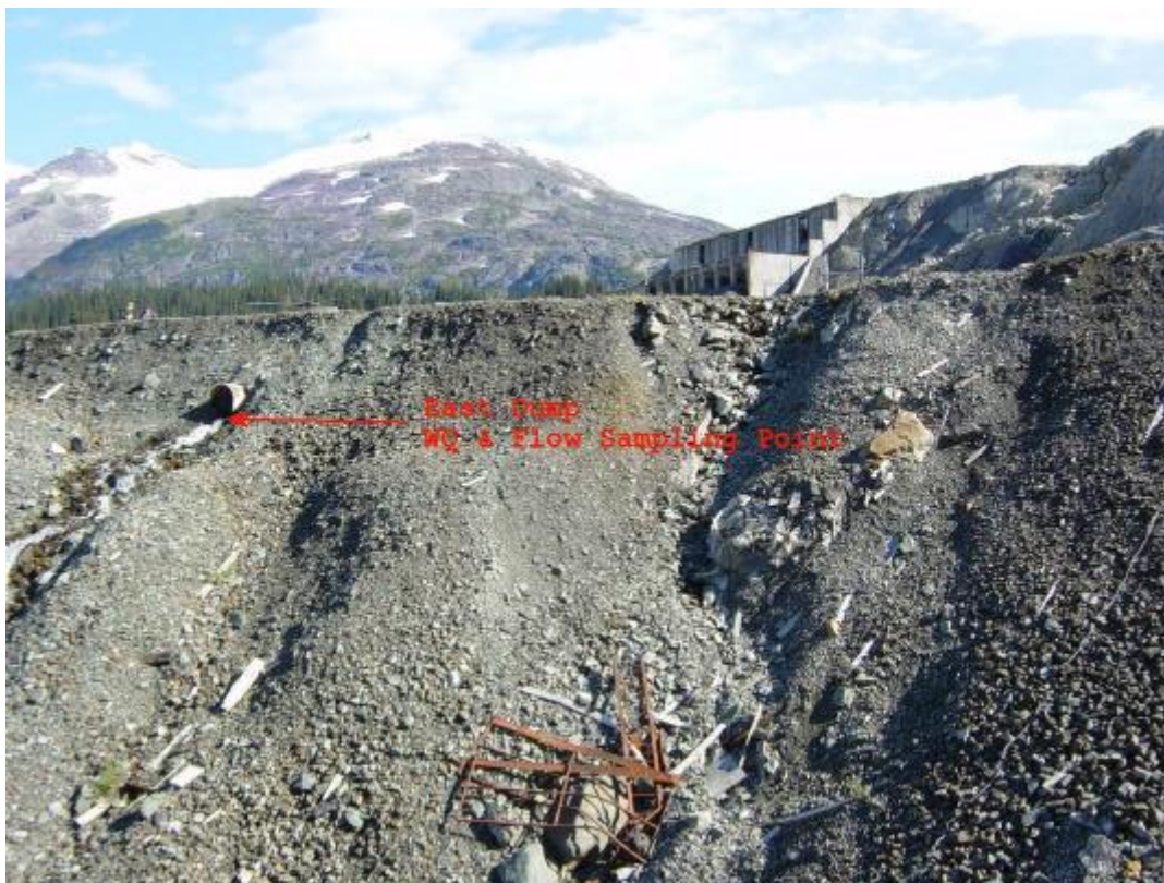
Figure 2: East Dump Culvert flow and water quality sampling location.
