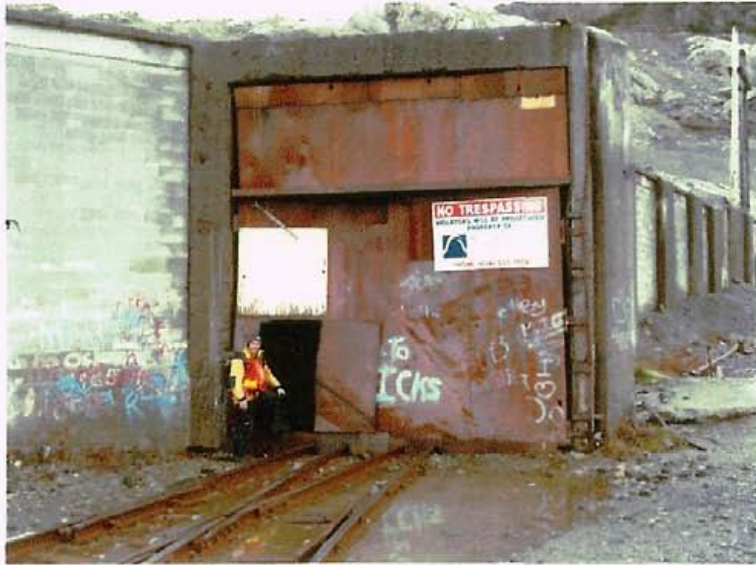
Photo-1 Entrance to the Gran Duc tunnel
