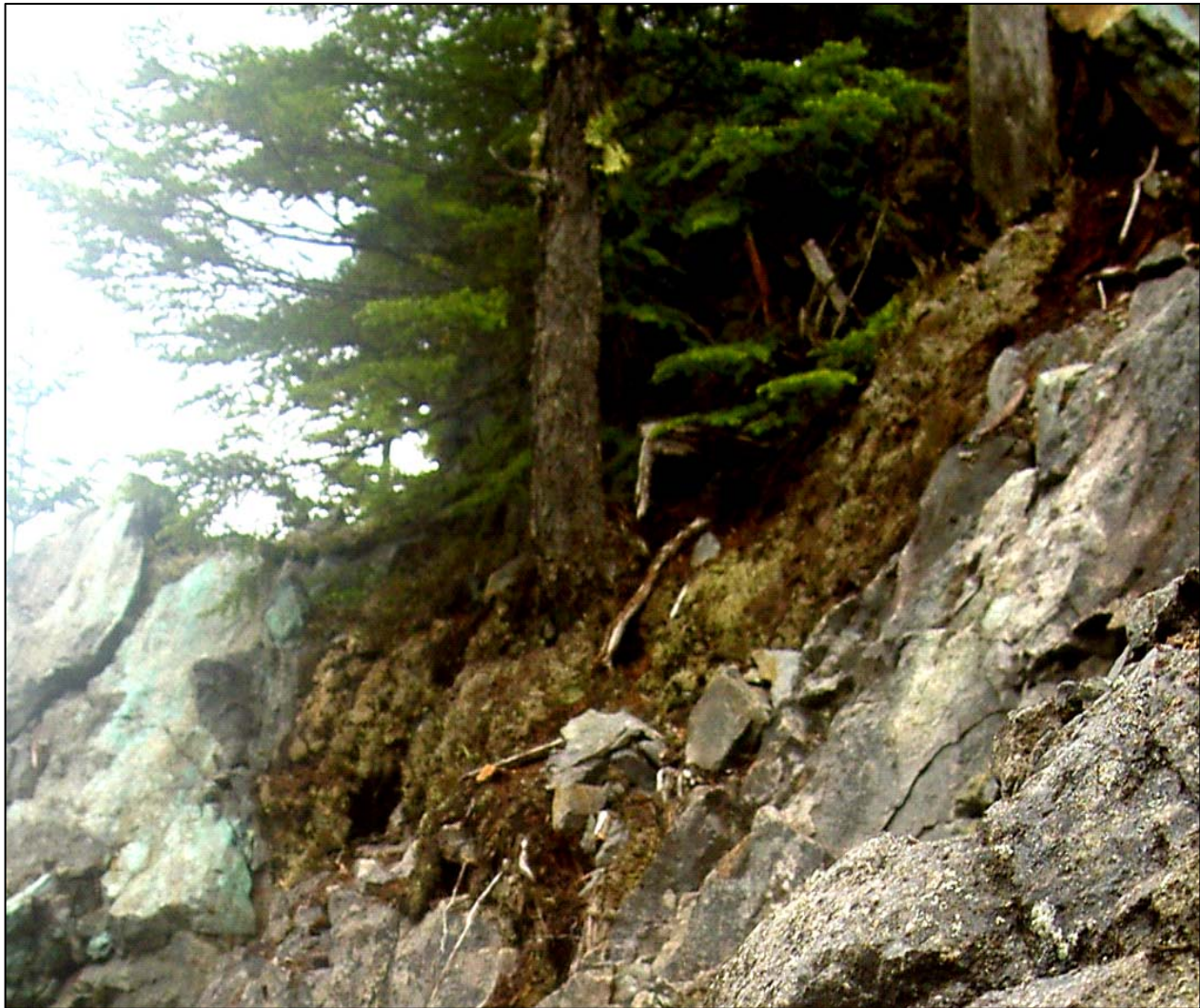
Figure 10: Downslope Mass Wasting at the Lucky Jim
