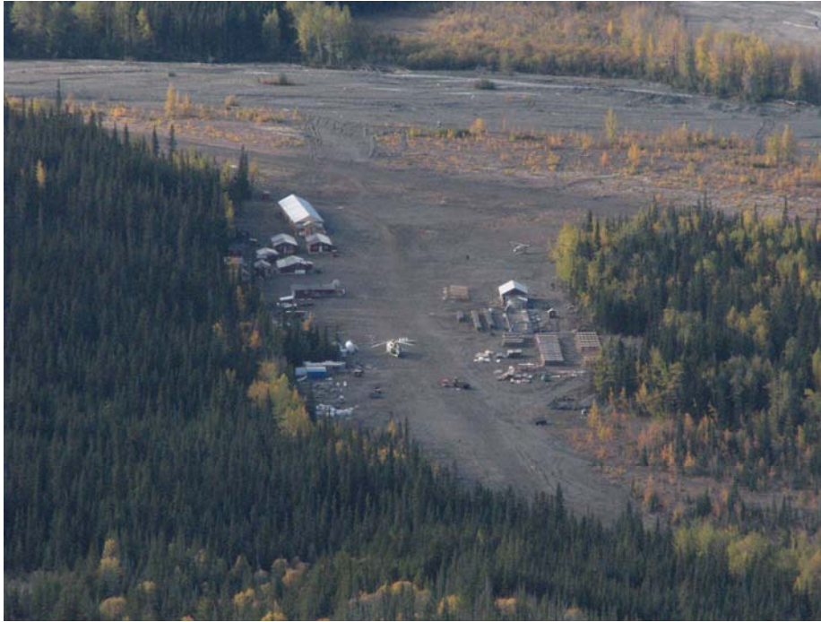
Figure 5-3. Camp facility 2007. Quanset buildings destroyed by high winter snowfall of 2006-07, conspicuously absent in this photo.
