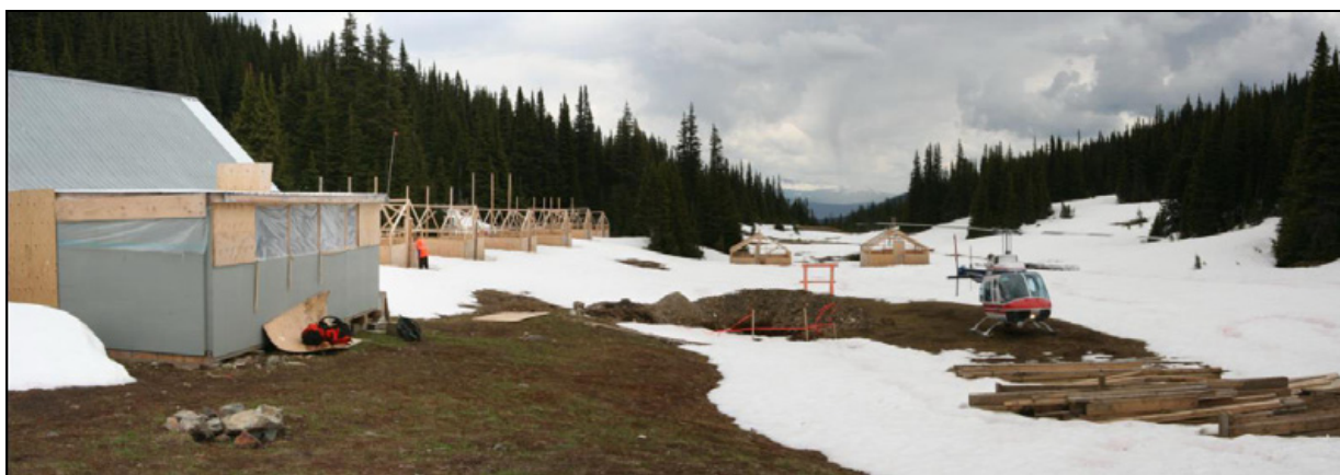
Figure 1.3. Geoinformatics' 2006 Field Camp in June 2007. All Structures Survived the Winter Intact
