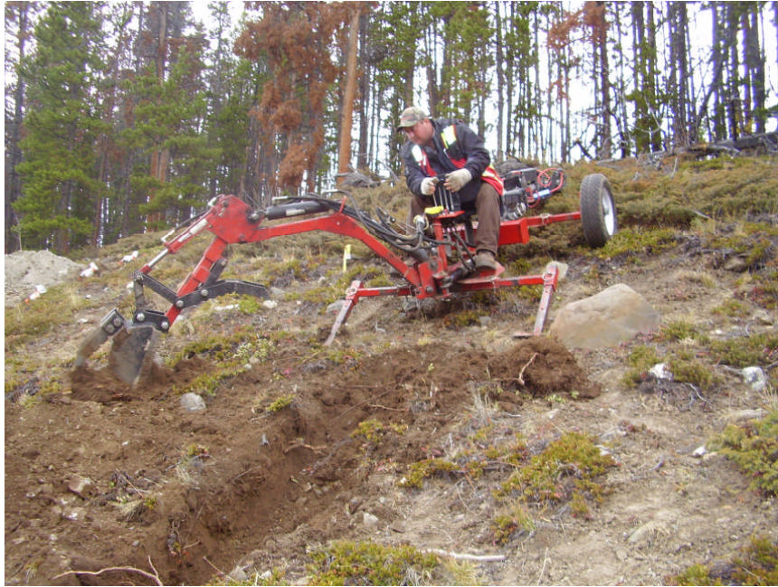
PLATE 1: Trenching on the Fame claims
