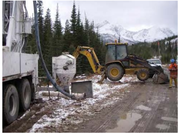
Photo 4: Cyclone setup on drill rig
