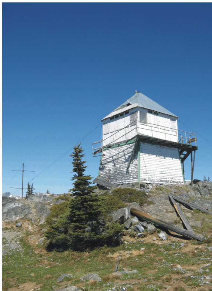
Figure 5. Abandoned fire tower, 1980m elevation, south of Botanie Mountain, Clear Range.
