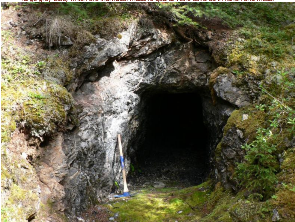
Picture 2. The entrance to the Wedge Project Adit dug in the 1930's. The Adit is ~8m long and extends into the side to the Wedge structure. (See Figure 5, Picture 5, and Map2)
