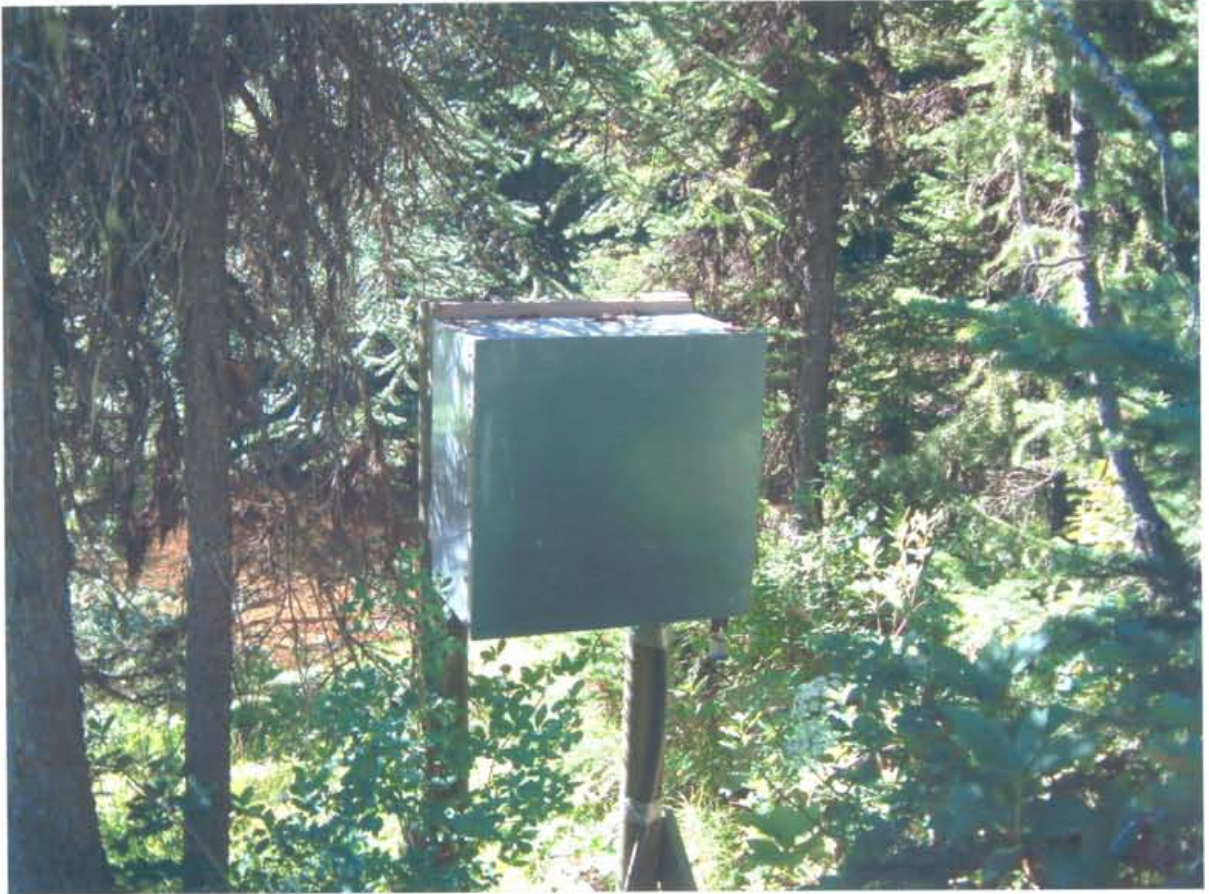
Baker Creek Hydrometric Station – Hydrologic Water Level Recorder Shelter
