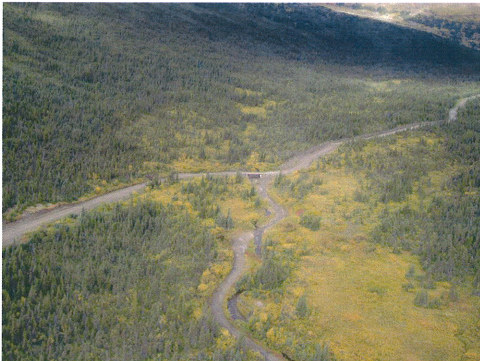
Picture 3 - West Logjam Ck Bridge
