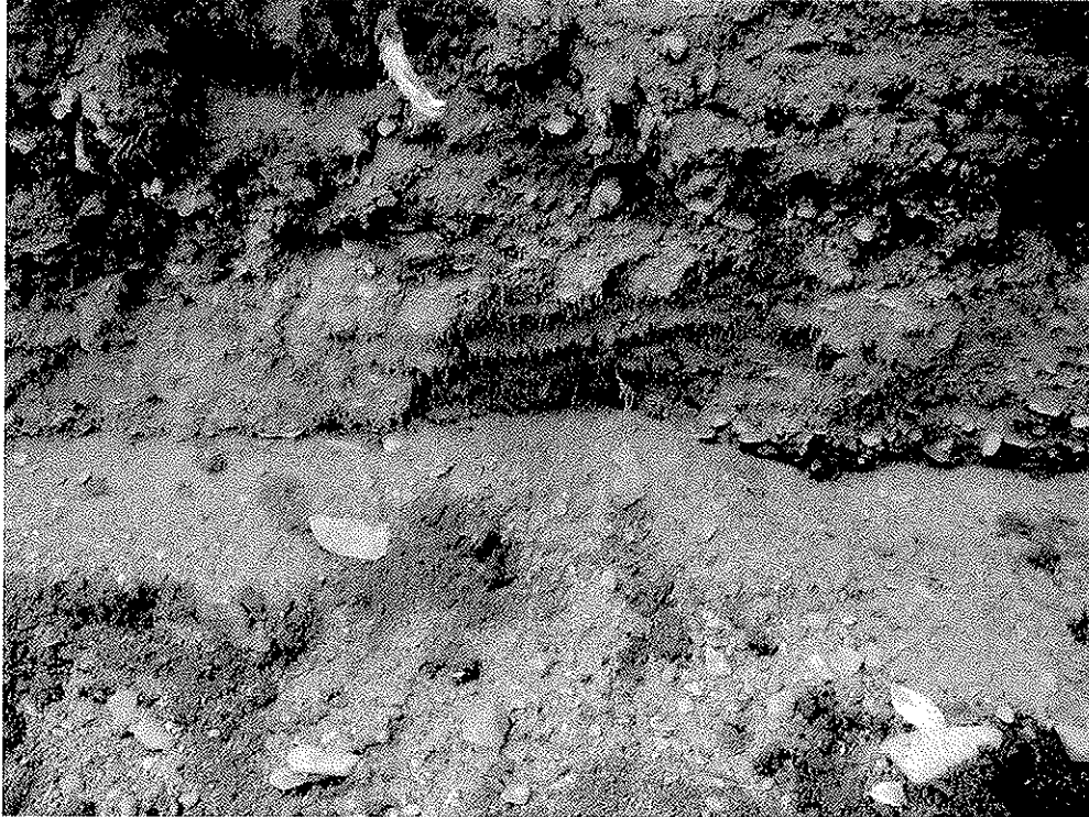
Picture 4 - Typical Sandy Gravel conditions
