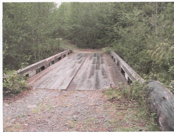
Parkinson Creek Bridge – WC-3000
