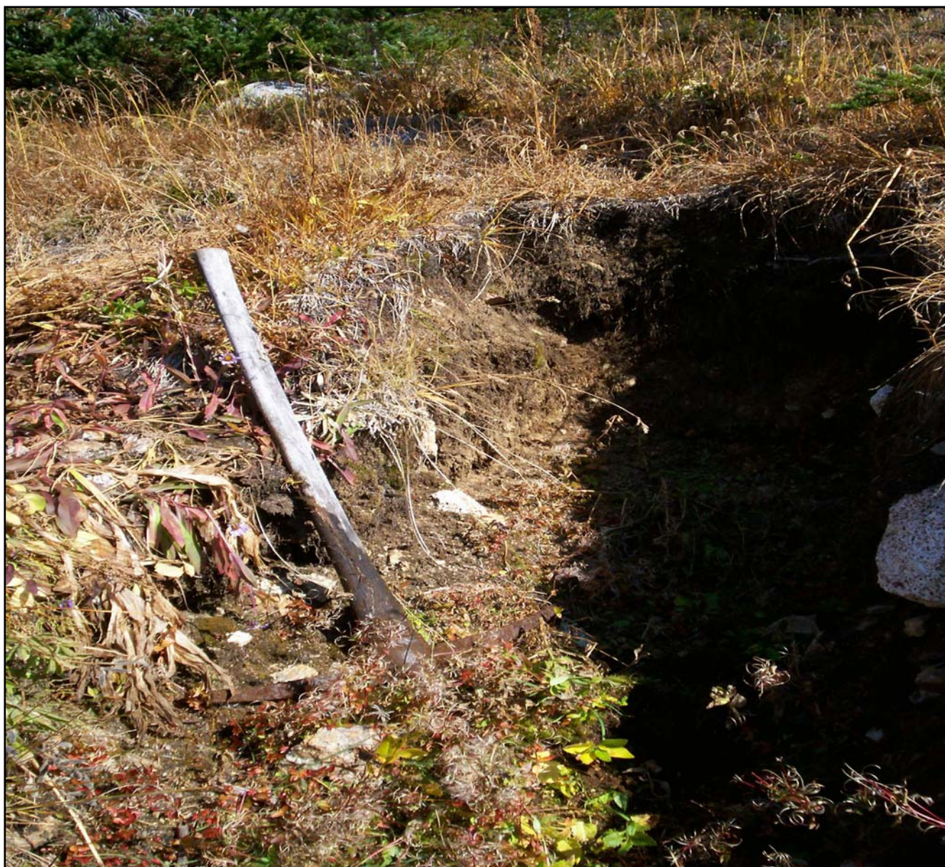
Picture 1:Trench with old Pick
