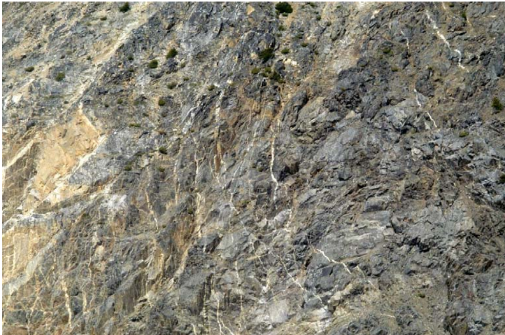
Figure 8: Quartz vein stockwork above access roads on east-facing slope of Molybdenum lake cirque ( ref. Fig. 12).
