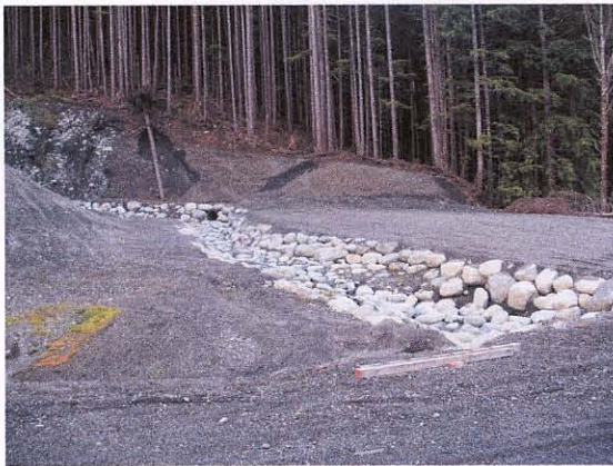
Sample sites – overburden and clay
