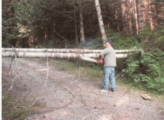
Tree removal – spur 10
