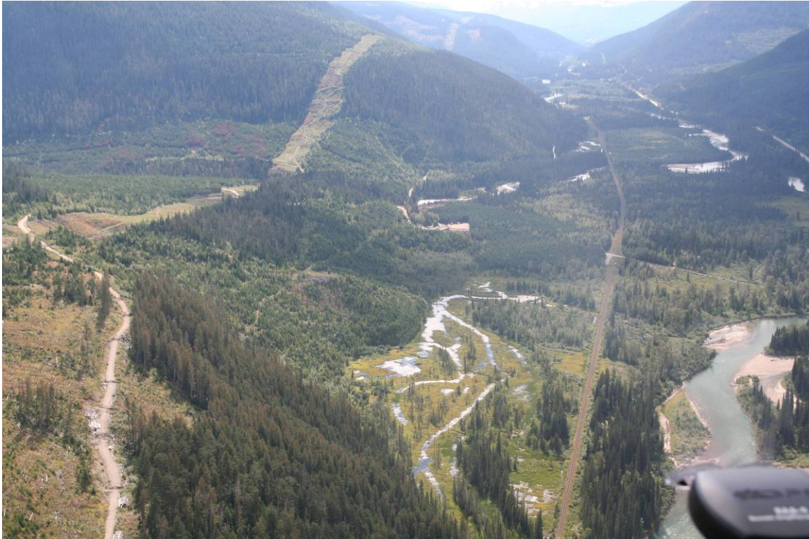
Figure 4 View of TSF4/WSF4 site showing swampy foundation conditions
