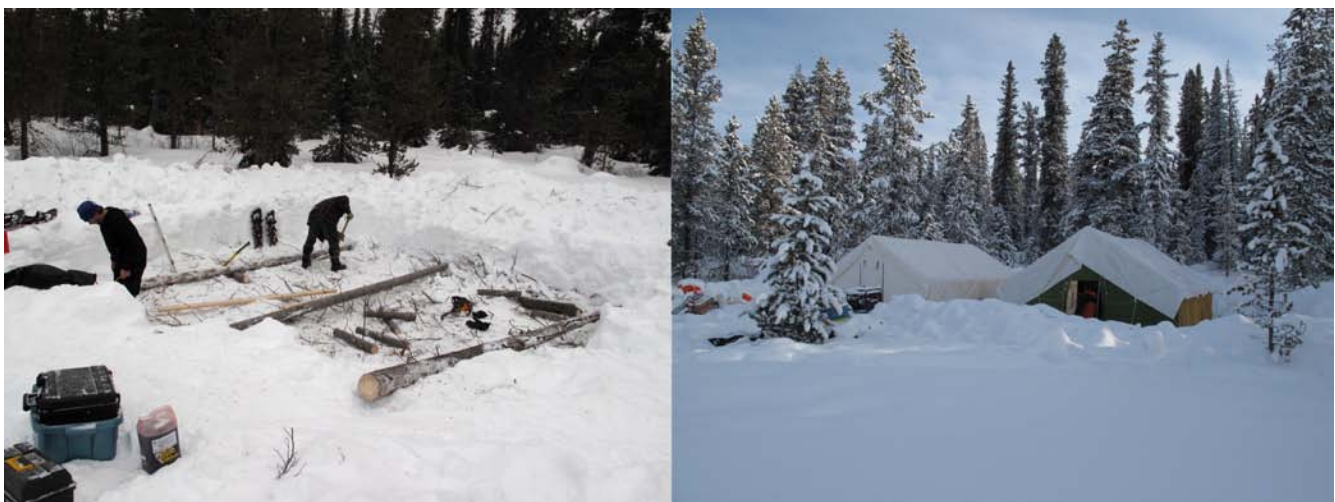
Figure 4: Pictures of camp construction (left) and final camp (right).
